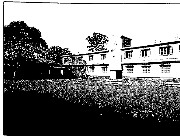
Constructing Girls' Hostel
